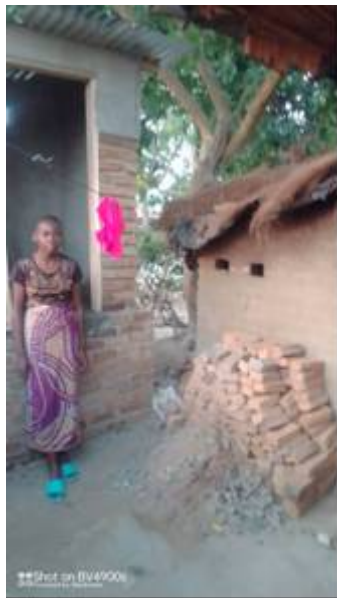
A new latrine being constructed for Precious Mwambira
