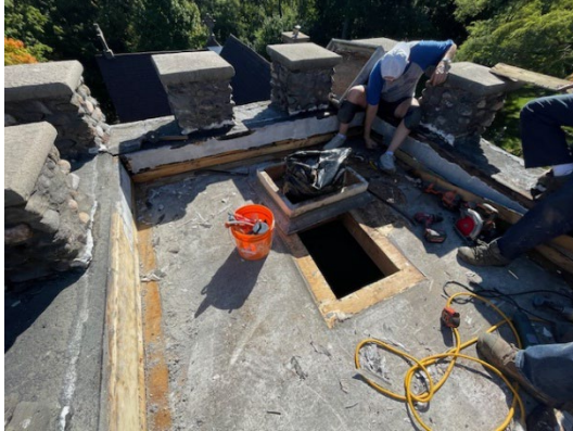
(removing the old roof)
